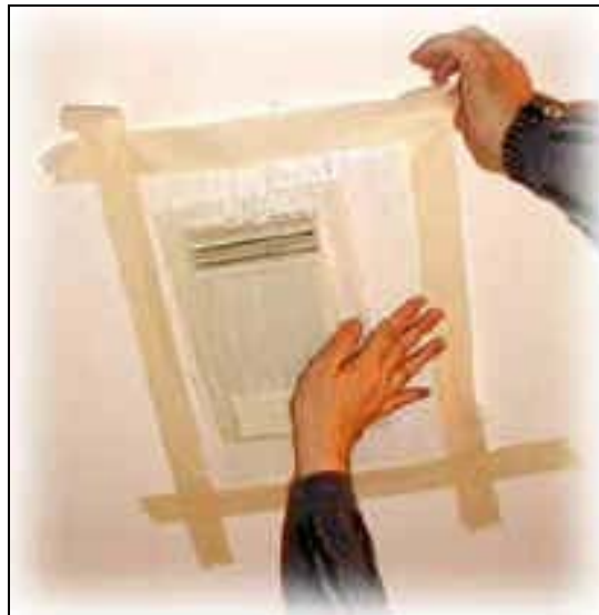
Sealing an Air Vent
