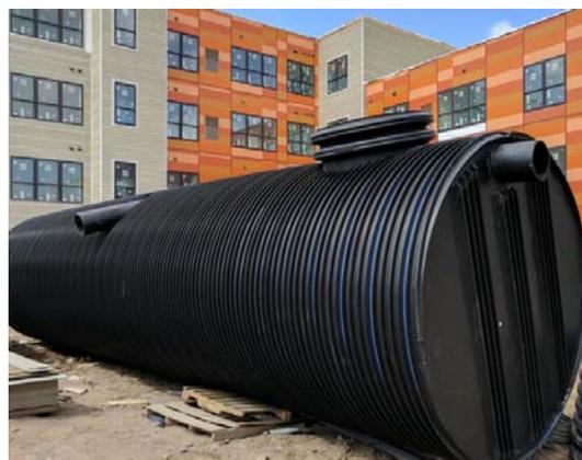
Figure 2: Stormwater Reuse Tank Prior to Installation at MWMO Capital Project Site
